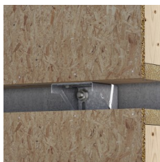
Brackets set below, on slab edge
